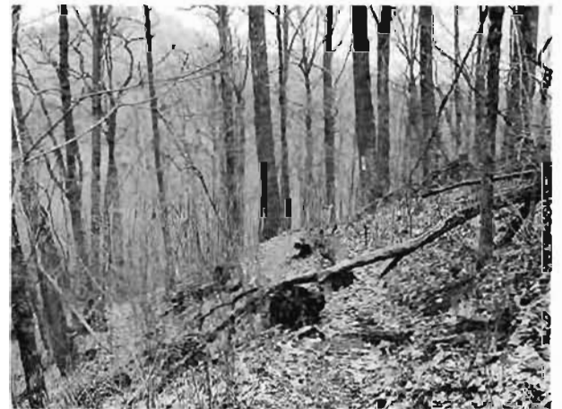
Fig. 2. Log barrier on sidehill slope, note white blaze (trail marker) in background
