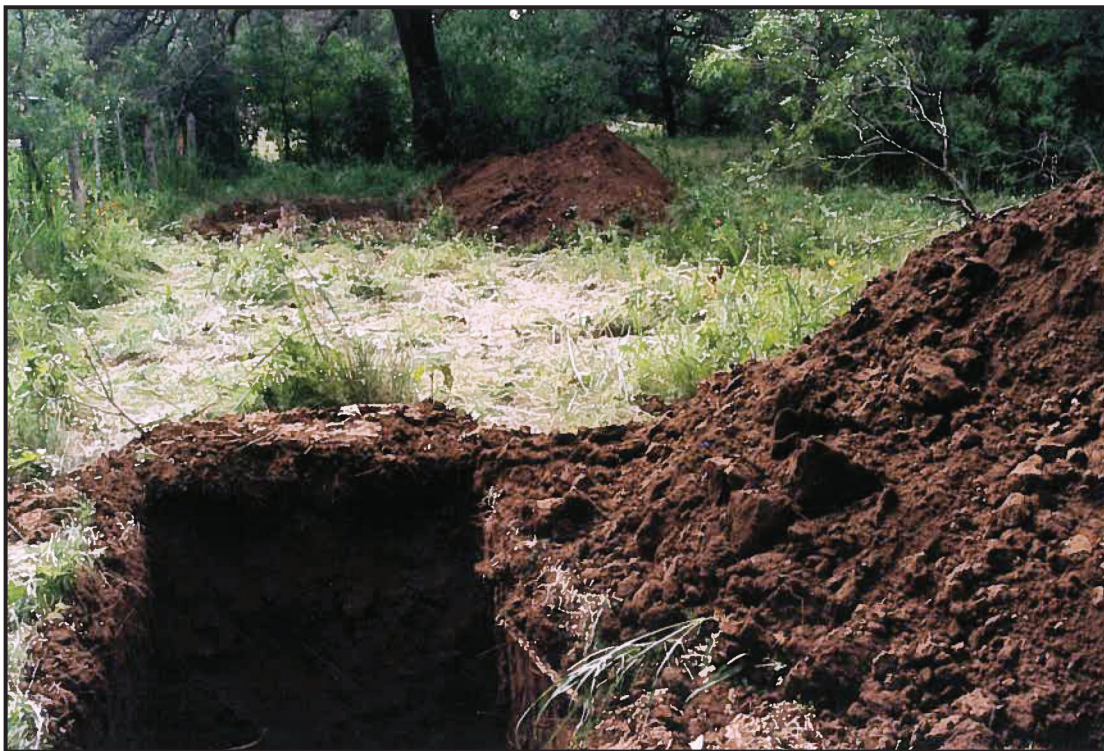
Figure 5-4. Excavated Backhoe Trenches 1 and 2 along right-of-way.
