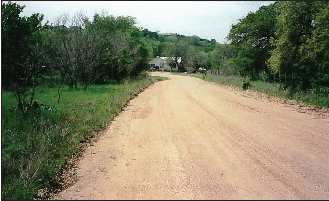
Figure 1-3. Existing roadway leading to old bridge.
