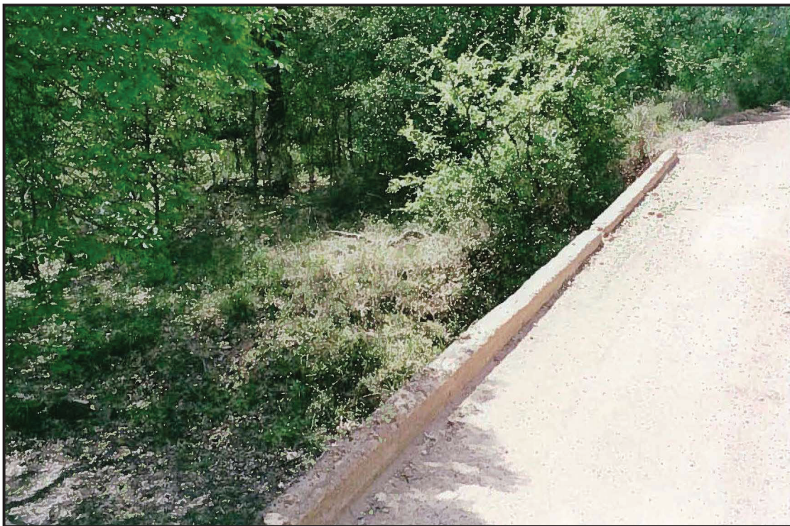
Figure 1-4. Edge of old bridge and surrounding vegetation.
